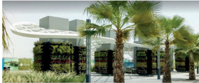
MASDAR CITY CENTRAL PARK LIGHTING PROJECT PHASE 2 ABU DHABI, UAE - 2022
