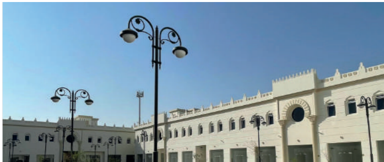
FARM HOUSE LANDSCAPE LIGHTING DOHA, QATAR - 2021
